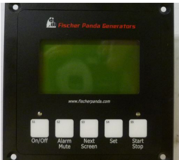
Generator control panel on the AC MDP
