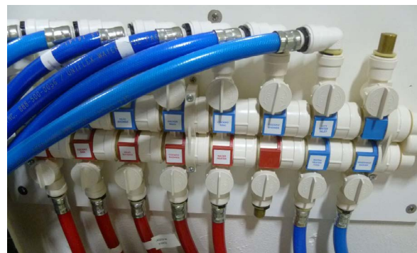
Water system manifold
