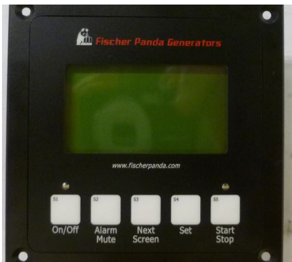
Generator control panel on the AC MDP
