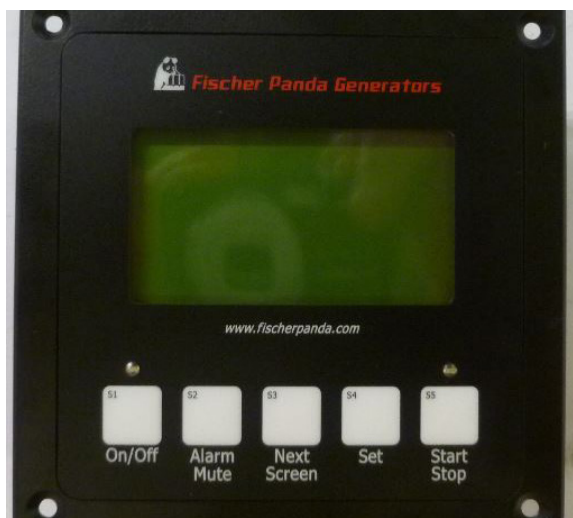
Generator control panel on the AC MDP
