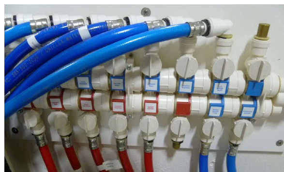
Water system manifold
