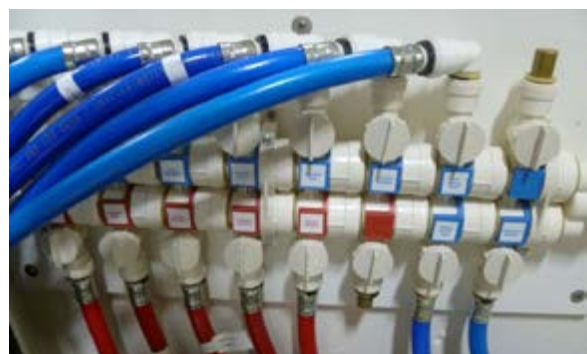
Water system manifold
