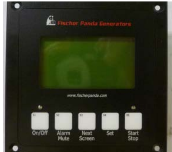
Generator control panel on the AC MDP
