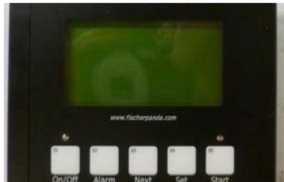
Generator control panel
