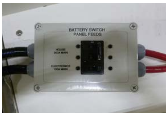
Battery switch panel feeds
