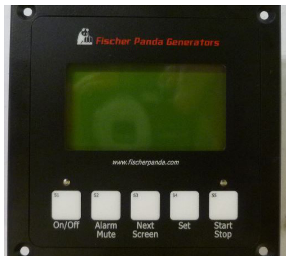
Generator control panel on the AC MDP
