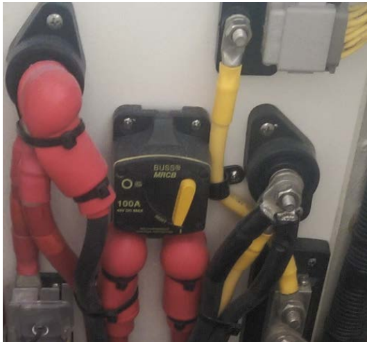
Main Battery Disconnect
